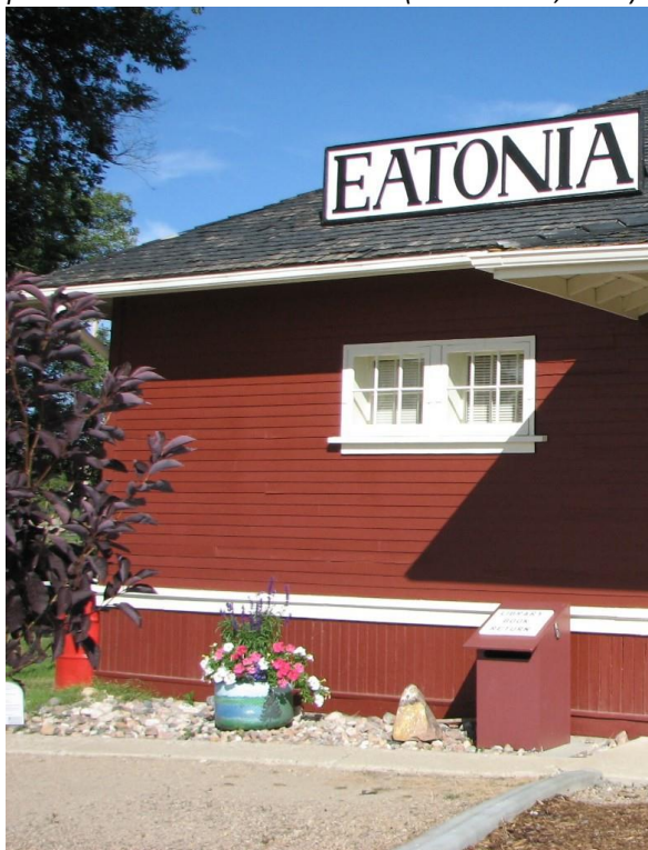
Fig.16 — The completed works demonstrate a high-degree of retention of the historic fabric (M. G. Miller, 2011)
