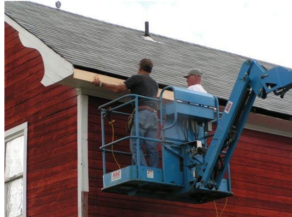
Fig. 8 — New materials, so long as they are in kind, will weather over time. Where new materials are required to correct constructional deficiencies, they should be compatible with the character of the place in terms of design and materiality (Photo: Village of Mortlach, 2009)
