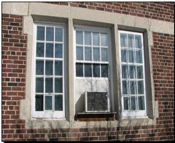
Diocese of Qu'Appelle complex, Regina SK Original storm windows feature numerous individual panes.
