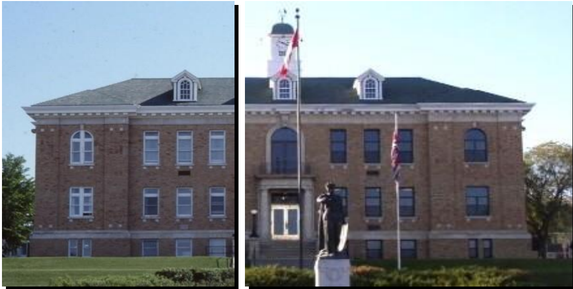
Court House, Prince Albert SK. - shown with the original white-framed wood windows (left) and the replacement black aluminum sealed units (right). Neither the colour nor the new window design replicates the original, thereby giving the building a very sombre appearance.
