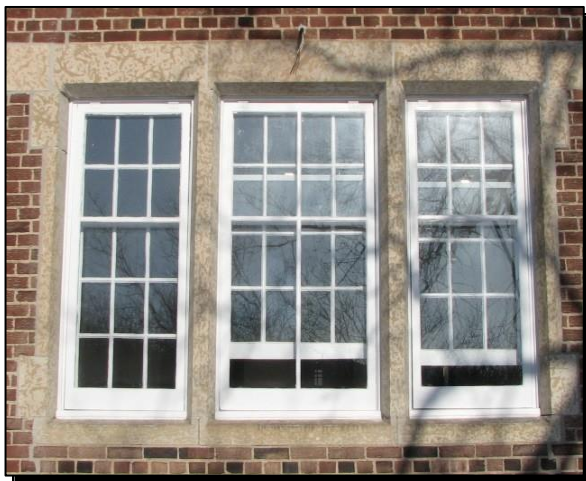
Diocese of Qu'Appelle complex, Regina SK Top-hung wood storm windows are acceptable. They protect historic multi-paned double-hung windows and can open.
