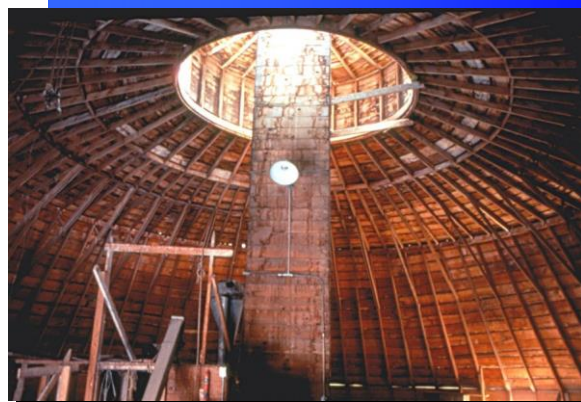
Termuende Barn Roof Interior, near Lanigan SK
