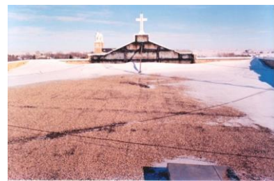
Elementary School, Gravelbourg Reroofing and parapet repairs
