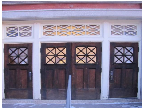
Fig. 11 —Melville City Hall, original character-defining doors and entrance (M. G. Miller, 2012)
