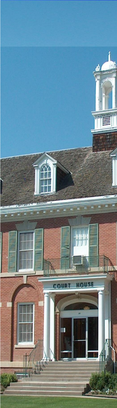
Fig. 19 — Weyburn Court House (above) —partial existing elevation showing front entrance (M. G. Miller, 2011)
