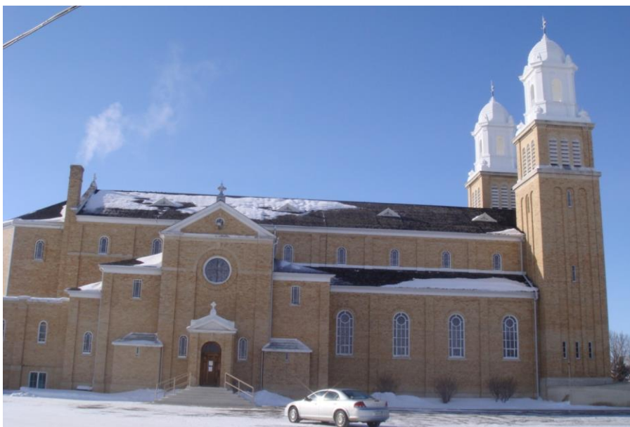
Fig. 21—The analysis of the historic mortar mix at the Co-Cathedral in Gravelbourg led to the selection of Type K mortar for its repointing.
