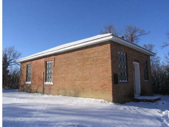
Fig. 1—The former Land Registry Office in Battleford was constructed in 1877-78. (Photo: M.G. Miller)
