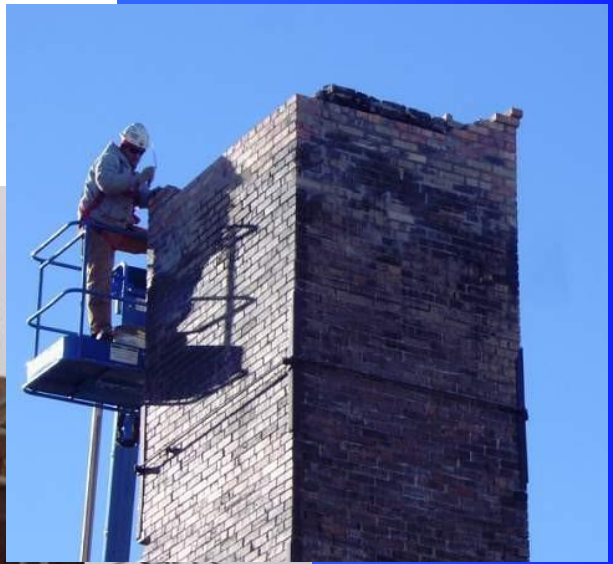
Fig. 25—Claybank Brick Plant NHS
