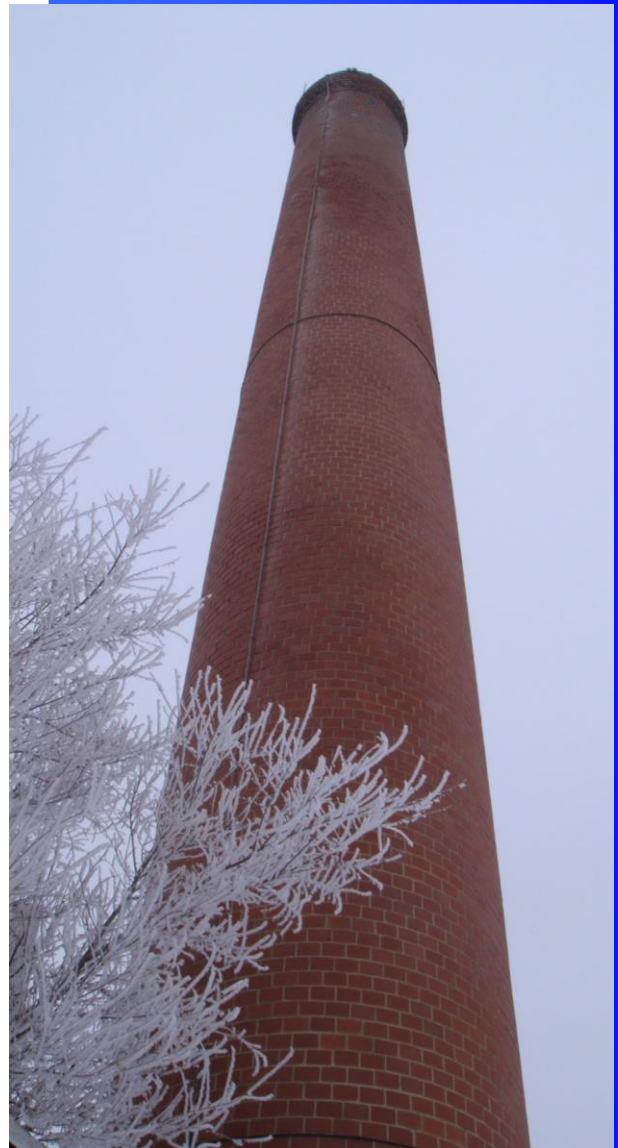
Fig. 5—The Soo Line Historical Museum, Weyburn, underwent masonry repointing in phases.
