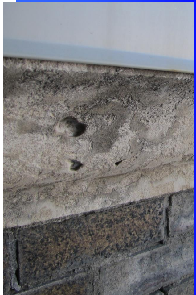
Fig. 16—Encrusted patina on the stone cornice at the former Land Titles Office in Moose Jaw.
