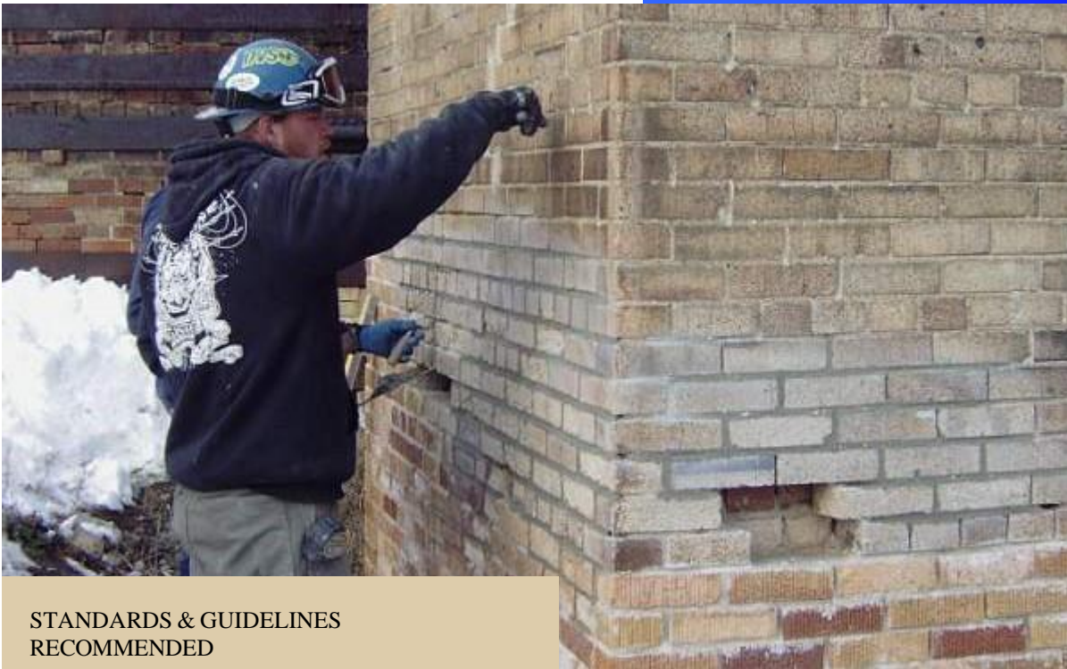
Fig. 24—Repointing the smoke stacks at Claybank Brick Plant NHS.
