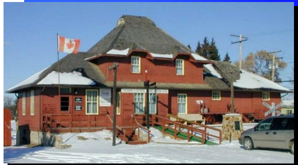
The former CPR Station at Theodore had to be relocated away from the railway tracks, and now serves the community as a local museum and drop-in centre.
