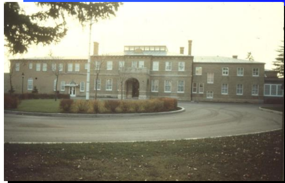
The restoration of Government House, Regina, in 1978-1980 included removal of an intrusive 1950s brick chimney and metal fire escape from the front of the building, but retention of the 1928 additions to the left and right of the original 1891 structure. However, new doors compatible with modern safety code requirements were installed in the primary entranceway at the left, while the original front doors, in the Romanesque-arched porte-cochere were retained and used only for ceremonial purposes.
